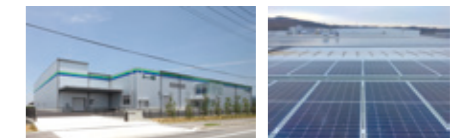
Installation of solar panels at ITO EN Kobe Factory (January 2023)
