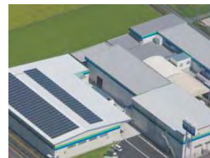
Solar panels installed on the rooftops of the facilities
