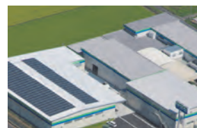
Solar panels installed on facility rooftop
