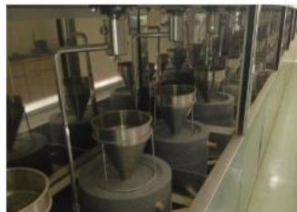
Dedicated matcha production plant (Shizuoka Factory)
